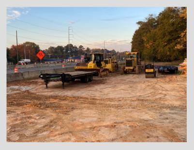
**SPLOST - Windy Hill Boulevard:** Baldwin has started the installation of storm drain on the southern side of Windy Hill. Baldwin has started building back the southern side drive lanes now installing GAB which is the second layer of roadway construction.
