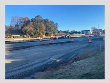
**SPLOST - Windy Hill Boulevard:** Baldwin has started the installation of storm drain on the southern side of Windy Hill. Baldwin has started building back the southern side drive lanes and installing GAB which is the second layer of roadway construction. They have also started installing sheet pile to start the southern side phase of the box culvert.
