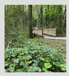
**Pedestrian Bridge Repair:** The pedestrian bridge at Tolleson Park was repaired by Quality Diversified Services. New handrails were installed across the bridge and some minor work was done on the underside to secure the bridge for park patrons safety.
