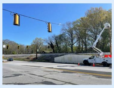
**Overhead Flashing Beacon – Riverview Road at Nichols Drive:** Mast arms were set on April 12th for an overhead flashing beacon at the intersection of Riverview Road and Nichols Drive. The overhead flasher was installed on Thursday, April 14th and is now active. This overhead flasher is intended to increase awareness of the all-way stop condition at the intersection.
