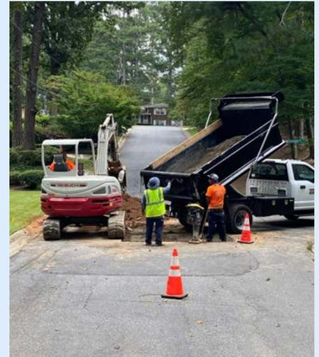
**Sewer Main Repairs:** Sewer crews dug up and repaired a collapsed sewer main on Rebecca Lane.
