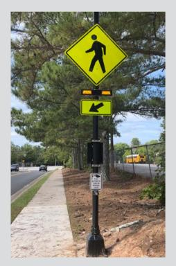
**Rectangular Rapid Flashing Beacon (RRFB) Installation:** A new solar-powered RRFB pedestrian crossing has been installed by the speed table near Campbell Road and Howell Drive at Campbell Middle School. This RRFB was installed by the developer of the Covenant United Methodist Church (located near the intersection of Atlanta Road and Campbell Road) in coordination with the Engineering Department.
