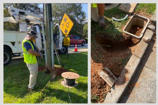
Traffic Loop Repairs: Our Traffic Signal Technicians are finalizing the traffic loop replacement at the intersection of Concord Road and Hurt Road. Once work is complete, we will begin replacing the setback loops at the intersection of Village Parkway and Lake Park Drive. The setback loops are needed for the approach on the mainline, heading northbound on Village Parkway.
