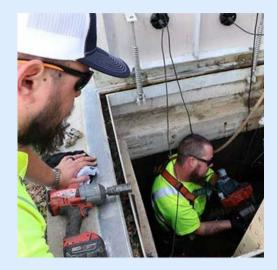
**Water Valve Maintenance:** Crews are performing valve maintenance in Ward 4 to ensure the valves are located and accessible. This maintenance reduces downtime and provides flushing of the system during water main breaks. While performing maintenance, crews are marking valves in the roadway with reflective markings to help staff locate valves when overnight emergencies arise. Projects will be ongoing through 2023.
