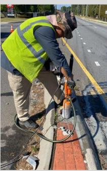
Windy Hill Road Signage: A series of one-way signs were replaced along Windy Hill Road between Village Parkway and Cobb Parkway. These signs are within the roadway median and are routinely hit by large trucks and errant vehicles.
