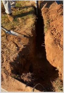
**Pedestrian Signal Repair:** Repairs are underway for the pedestrian signal that was struck during a traffic accident at South Cobb Drive and Powder Springs Street. The original signal was pole-mounted and will now be mounted on a signal post. Our Traffic Signal Technicians ran new wire from the traffic signal pole and poured the concrete foundation in preparation for the new signal post installation.
