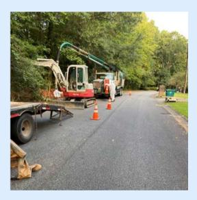
**Outfall Lines:** Staff is inspecting and clearing outfall lines around the city. Outfall lines are what connect sewers to subdivisions and streets so sewage can exit to the sewage plant downstream.
