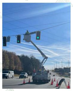
**South Cobb Drive/SR 180 Street Name Sign Updates:** The last intersection for phase 1 of the street sign updates is complete. Our Traffic Signal Technicians replaced the street name signs at the signalized intersection of South Cobb Drive and Cooper Lake Road, which were last installed in 2007. The next phase of street name sign updates will include the southern section of SR 280 stretching from Ridge Road to River View Road/Maner Road.
