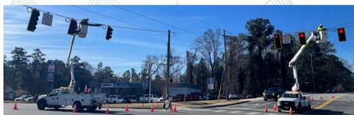
Concord Road Signs: Our Traffic Signal Technicians have assisted with the Concord Road median project by installing a series of signs (including traffic calming ahead, dynamic speed display, and keep right median signs), and are currently working to install the pedestrian assembly and rectangular rapid-flashing beacon for the mid-block crossing near Concord Road and Highview Drive. The base for the assembly is set with the remainder of the assembly scheduled for installation next week.
